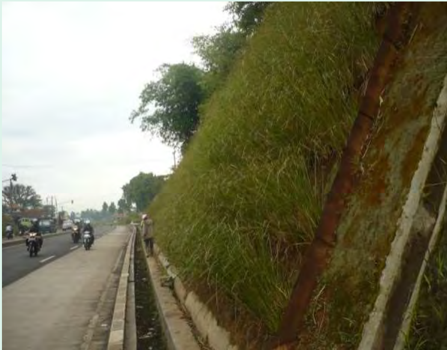
Slope 80°, Age: 4 months Before trimming
