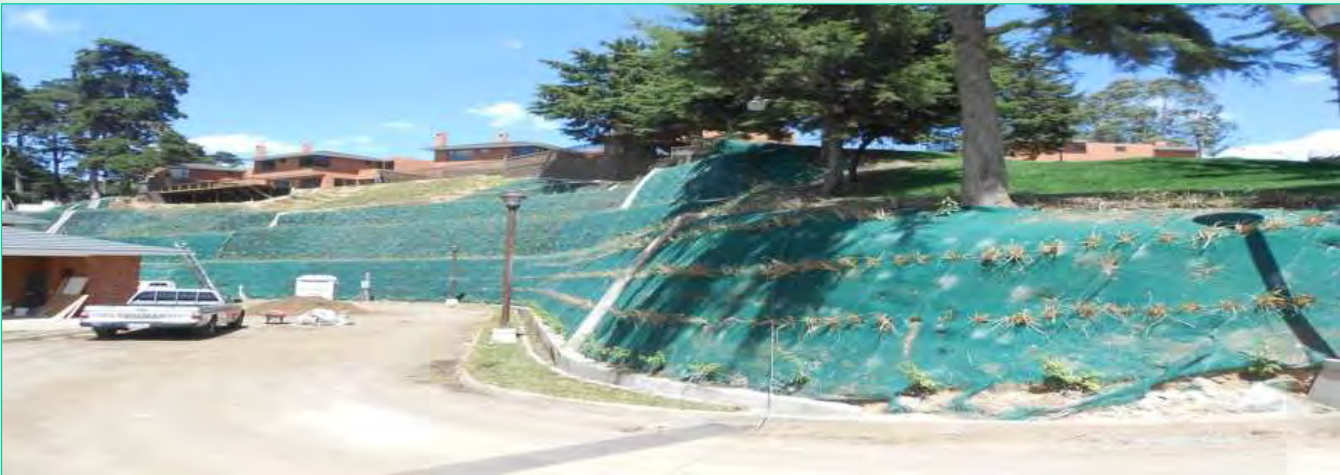
Very steep batters with geofabrics
