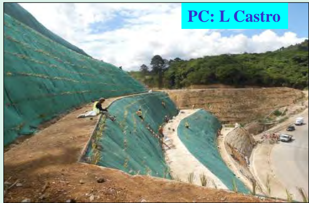
Very steep batters with geofabrics
