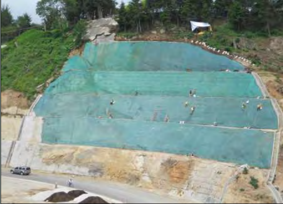
Very steep batters with geofabrics
